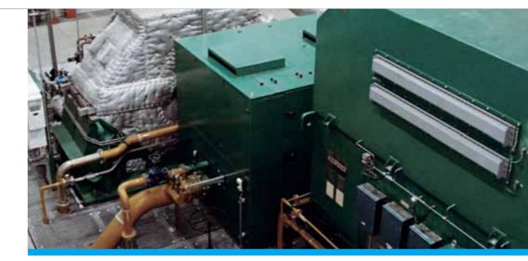
In industrial steam turbines, portions of the available steam are often extracted for production purposes, heating steam networks or for regenerative feed water heating. In addition to multiple bleed ports, controlled extraction can also be provided. The MARC® series allows turbine components to be optimally designed to meet individual requirements based on pressure levels and extraction volumes.
